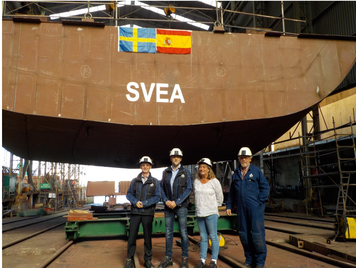
Photo taken at the time of the official keel laying.
